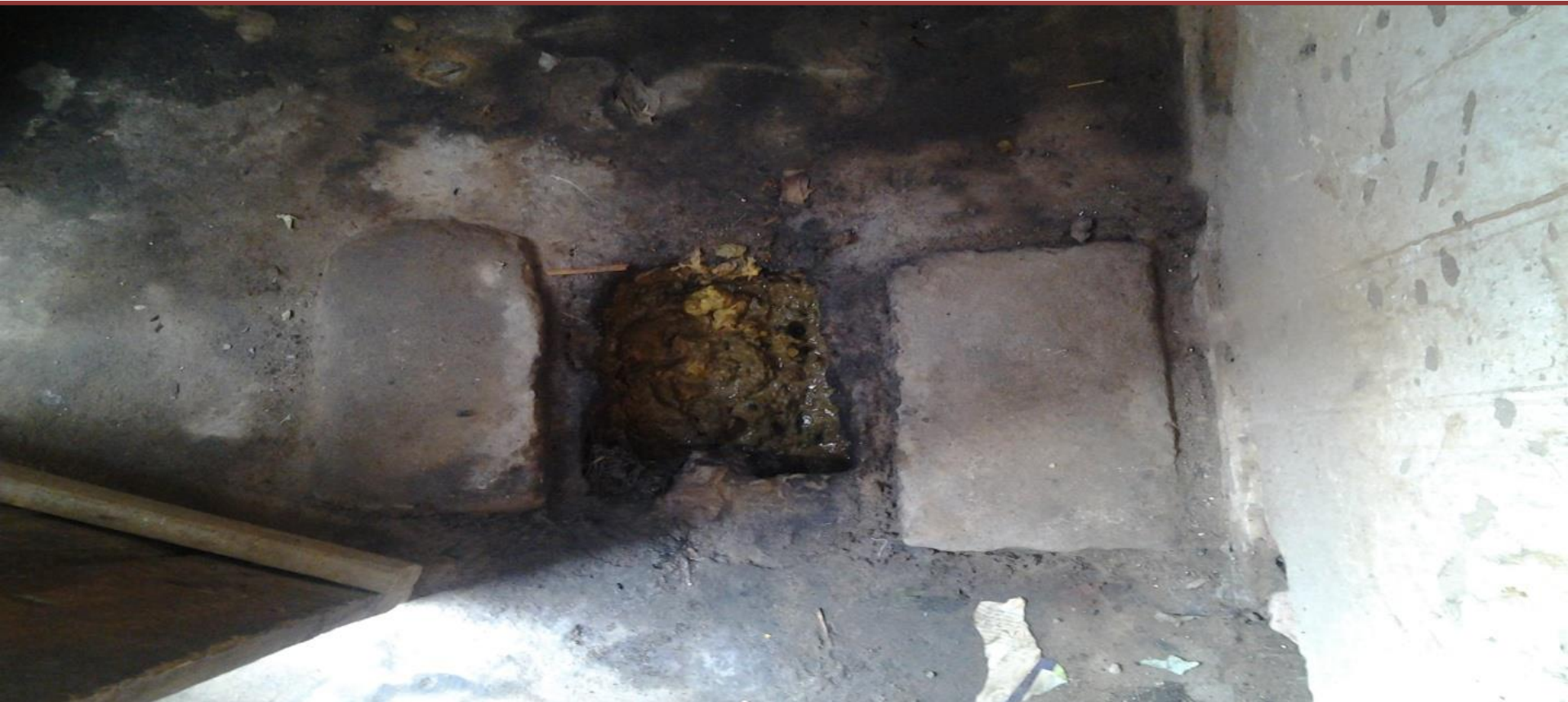
Figure 4: An Aerial view of a full pit latrine at Chiputula Township, an informal settlement within Mzuzu city Photo: Chipeta, 2014
