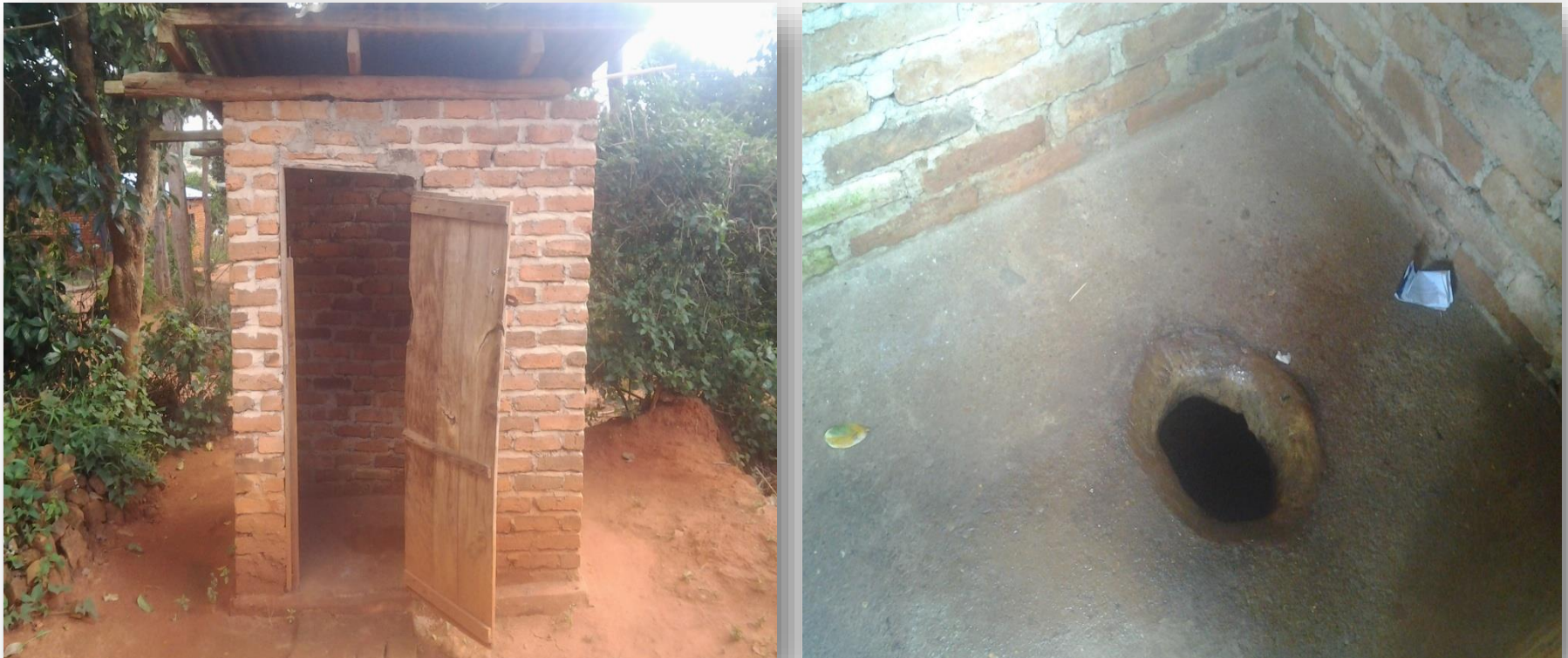
Figure 1: Pit Latrine in Luwinga , Mzuzu, Malawi Photo: Chipeta 2014
