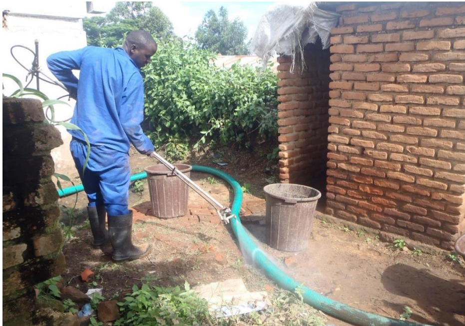
Water jet employed for cleaning also utilised for agitating hard sludge
