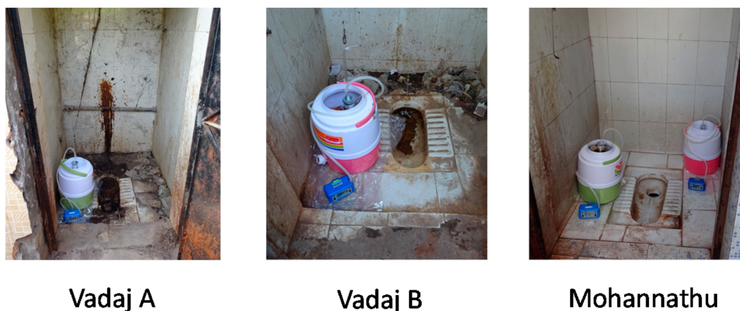
Figure 4. Latrines analyzed in India. Ahmadabad Khada Vadaj and Ahmadabad Behrampura, Mohannathu. In Mohannathu, two identical samplings were performed.
