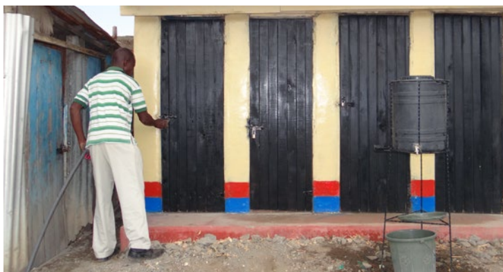
One of the toilets constructed under the UBSUP programme.
