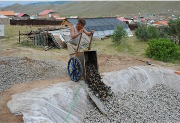
Figure 23: Screening (top left), loading (bottom left) and cleaning of the gravel during construction & assembling of the distribution system with holes (top right) (ACF, 2013).
