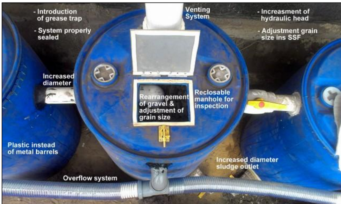
Figure 29: Visualization of the technical adjustments applied at the GHTU (ACF, 2013).
