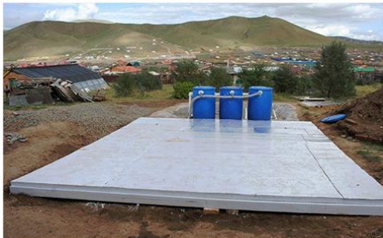
Figure 39: Pictures from the IBU. Covered storage pond in front, septic tanks behind and CW in the back (left). Covered collecting chamber in the front, CW behind, septic tanks left (right) (ACF, 2013).
