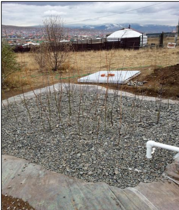
Figure 19: Photo of the VFB constructed wetland planted with willow at the IBU (ACF, 2013).
