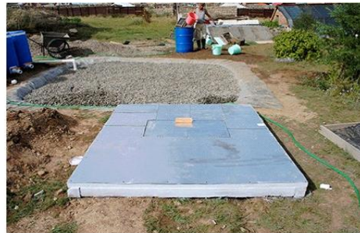
Figure 39: Pictures from the IBU. Covered storage pond in front, septic tanks behind and CW in the back (left). Covered collecting chamber in the front, CW behind, septic tanks left (right) (ACF, 2013).
