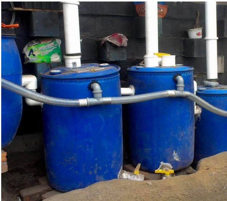
Figure 15: Septic tank at the GHTU during construction (ACF, 2013).
