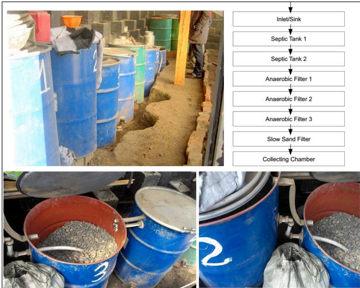
Figure 27: Photos of the IGHU (built in 2010) with technical shortcomings and flow chart (ACF, 2012; modified by Schüssler, 2010).
