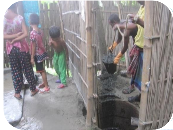
Lack of capacity in collection and transportation of sludge
