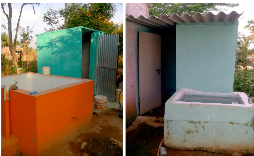
Tanks with piped water facility near NBA toilets in Dharmapuri, Tamil Nadu [Tank portion not a part of the NBA design or incentive].
