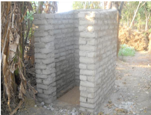
(1) Half built NBA Toilet – contractor/NGO built (Odisha)
