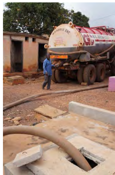
Emptying a public septic tank in Bantama Photo credit: Claire Furlong
