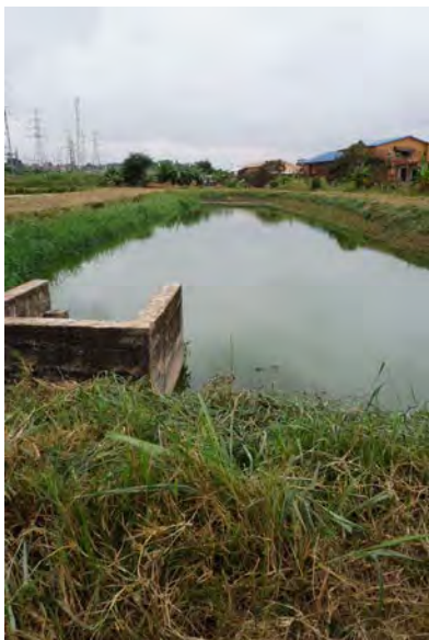
Maturation pond at Asafo Sewage Treatment Plant Photo credit: Claire Furlong
