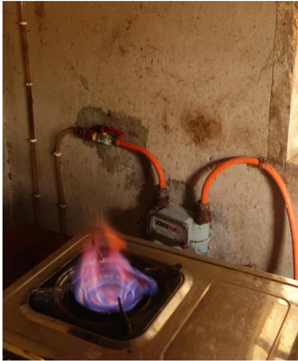
Biogas used for cooking. Photo credit: Imanol Zabaleta
