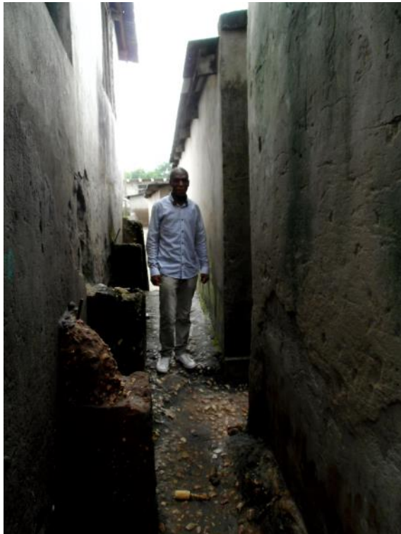
Path inaccessible to vacuum trucks
