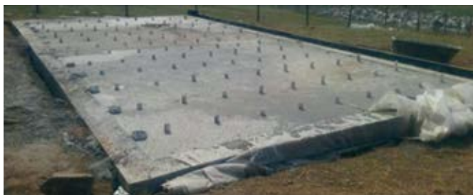
PHOTO 15: PASSIVE AERATED PLATFORM DURING CONSTRUCTION.
