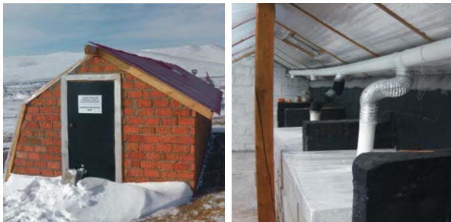
PHOTO 14: GREEN HOUSE UNIT OUTSIDE (LEFT) AND INSIDE (RIGHT). SOURCE: ACF.
