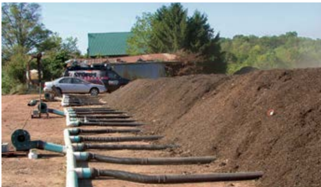
PHOTO 5: AERATED STATIC PILE. SOURCE: [62]
