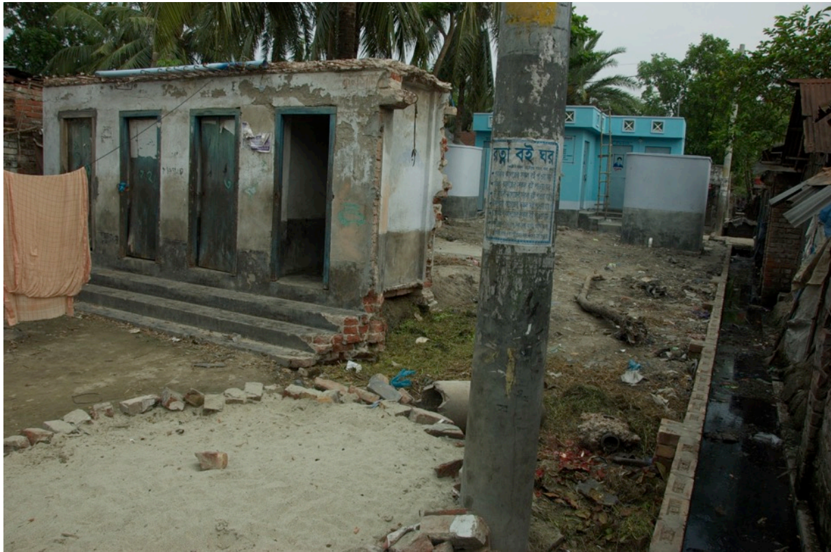
Figure 2: Abandoned community toilet (front) and newly constructed community toilet (back) in the low-income area of Bastuhara. Open drain on the right. Photo: Lars Schoebitz
