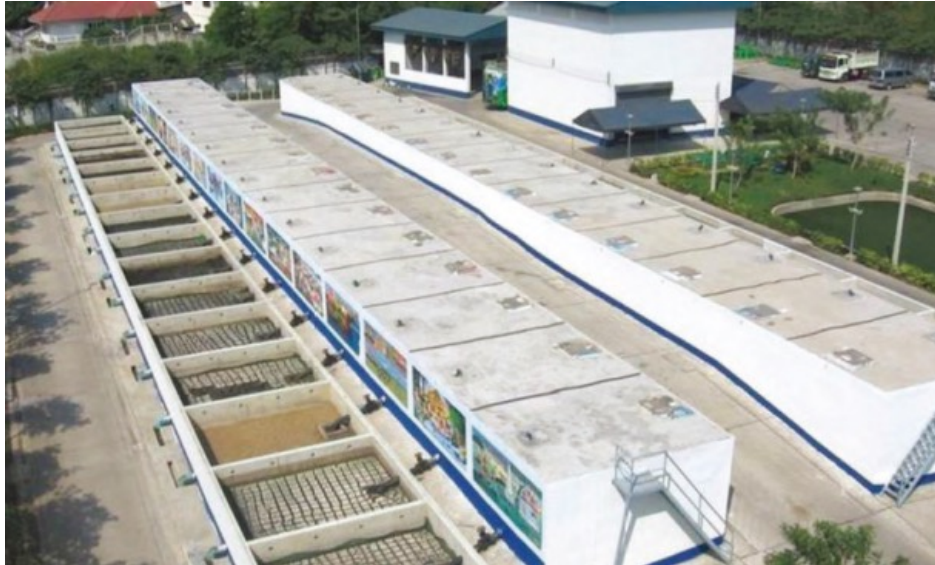
Figure 5: The bio-fertilizer plant, a faecal sludge treatment plant of Nonthaburi City Municipality (1). AECOM & Eawag/Sandec (2010)
