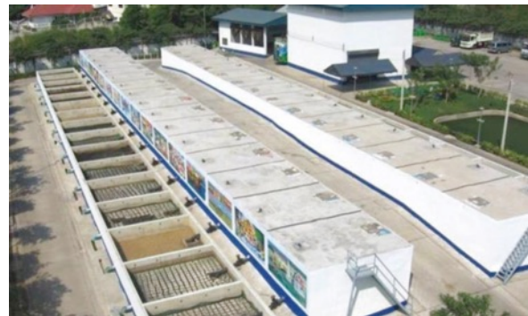
Figure 1: A faecal sludge treatment plant of Nonthaburi city, called the bio-fertilizer plant (Source: AECOM & Eawag/Sandec 2010)
