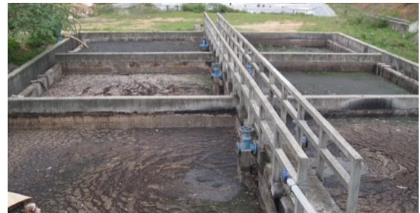
Figure 1: A faecal sludge treatment plant of the Khanh Son Landfill (Source: Hidenori Harada/Kyoto Univ. 2009)
