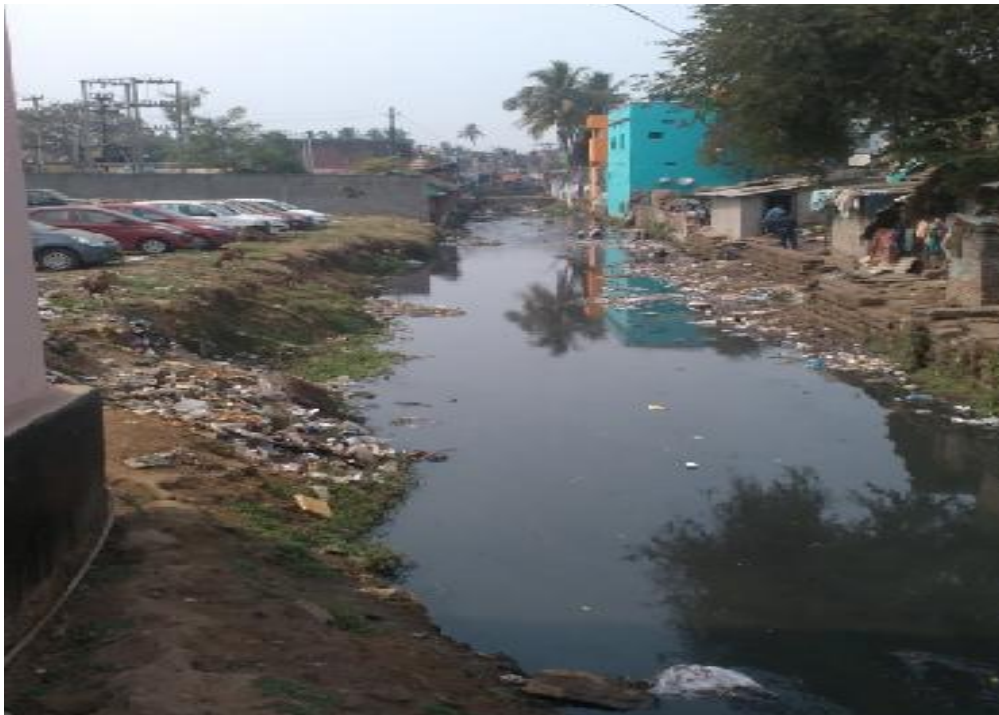
Figure 3: Open drain carrying sewage
