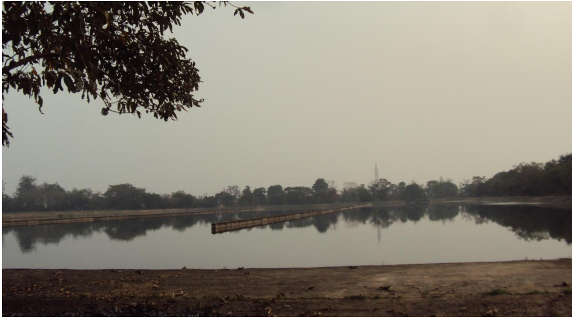
Figure 5: Waste stabilization pond
