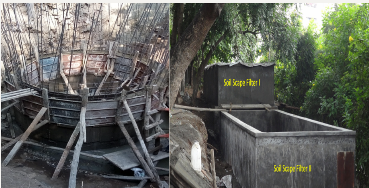
Figure 6 - Construction of intake well (left) and soil scape filter beds (right).
