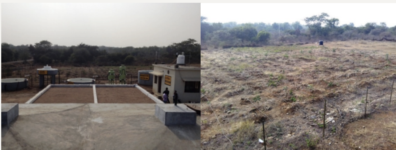
Figure 3: Aerial view on the vertical –up-flow constructed wetlands of the main treatment line (before plantation, left) and short rotation plantation (SRP, right) at OFAJ Site, Nagpur
