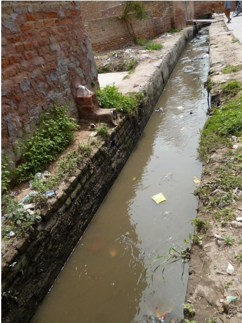
Figure 5: Open drain(Source: Rahul/CSE, 2015)
