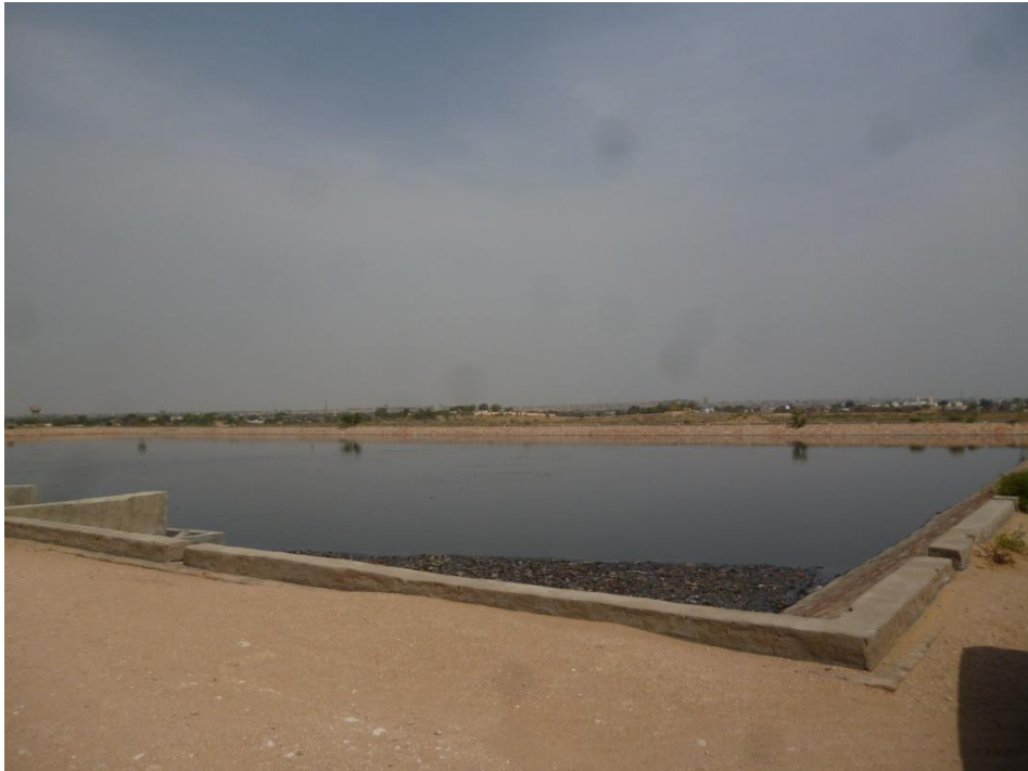
Figure 8: Waste Stabilization Pond in Vallabh garden (Source: Shantanu/CSE, 2015)
