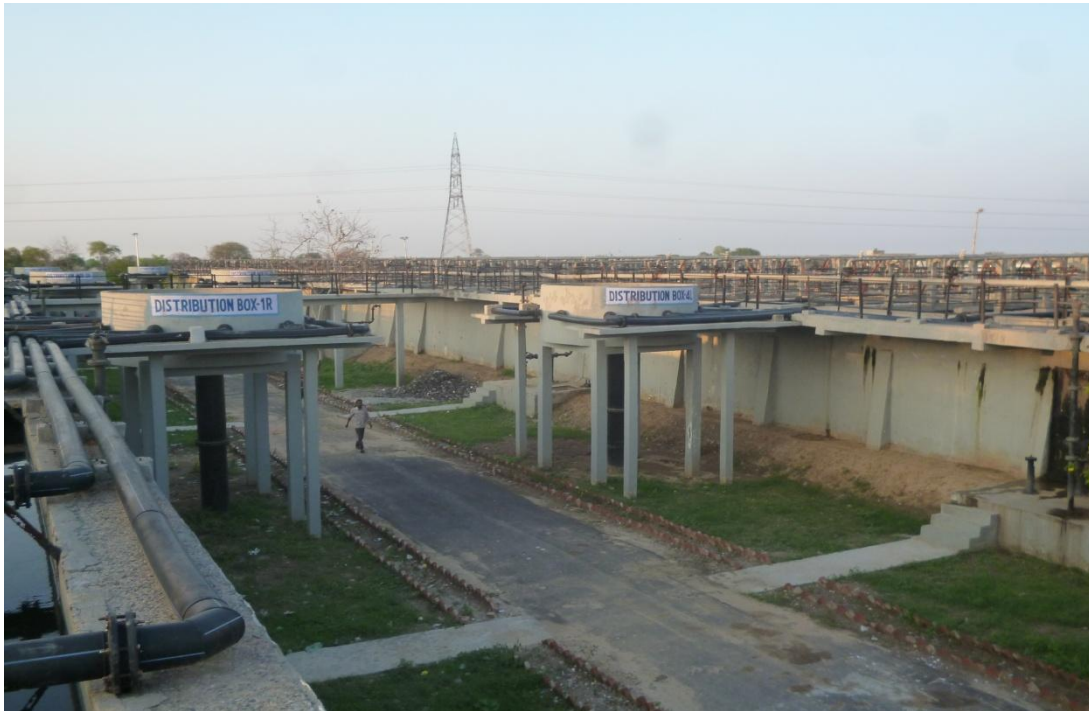
Figure 5: 78 MLD UASB technology Dhandpura STP (Source: Shantanu/CSE, 2015)
