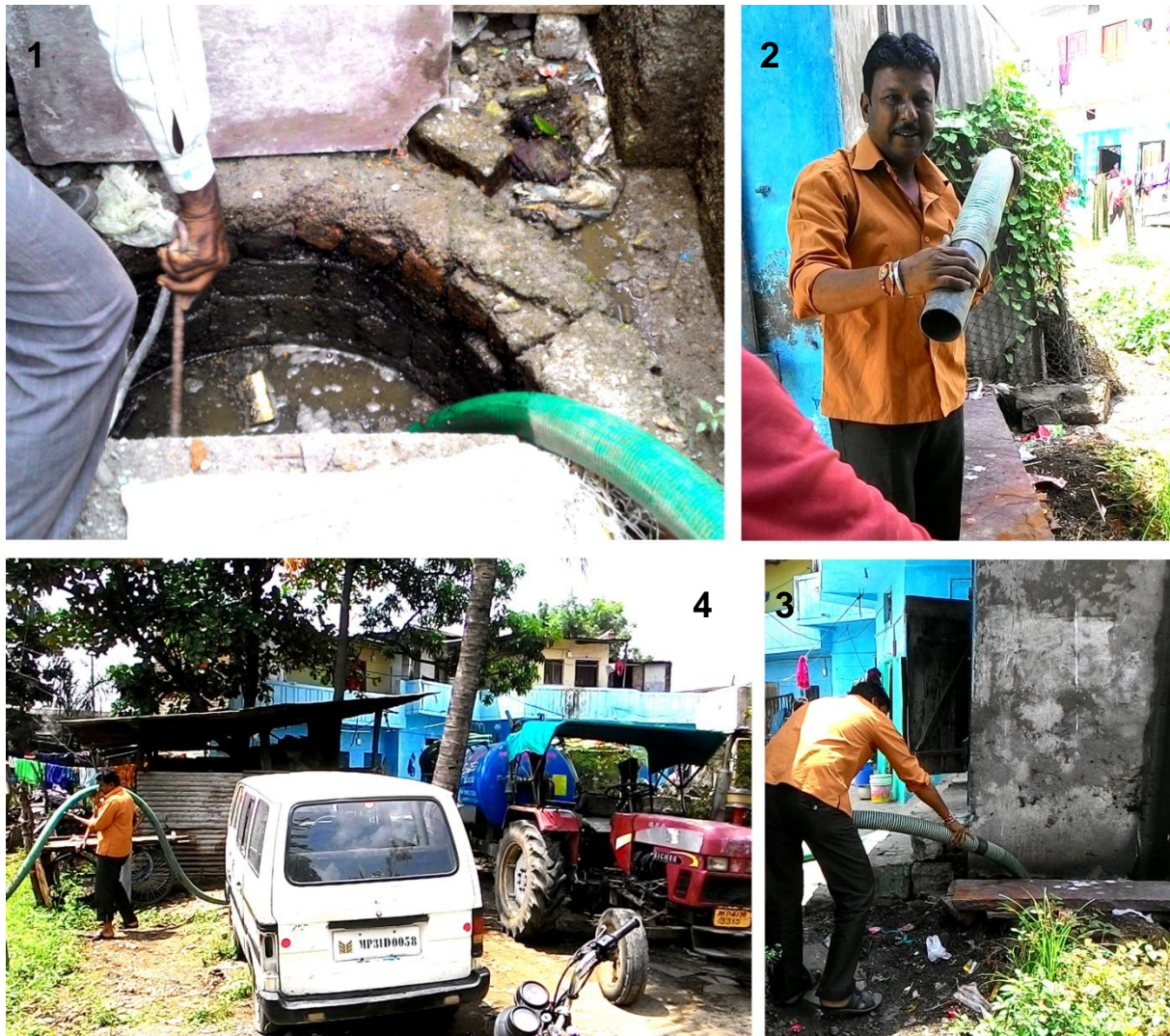
Figure 7: Emptying service by DMC (Source: Rahul/CSE, 2015)
