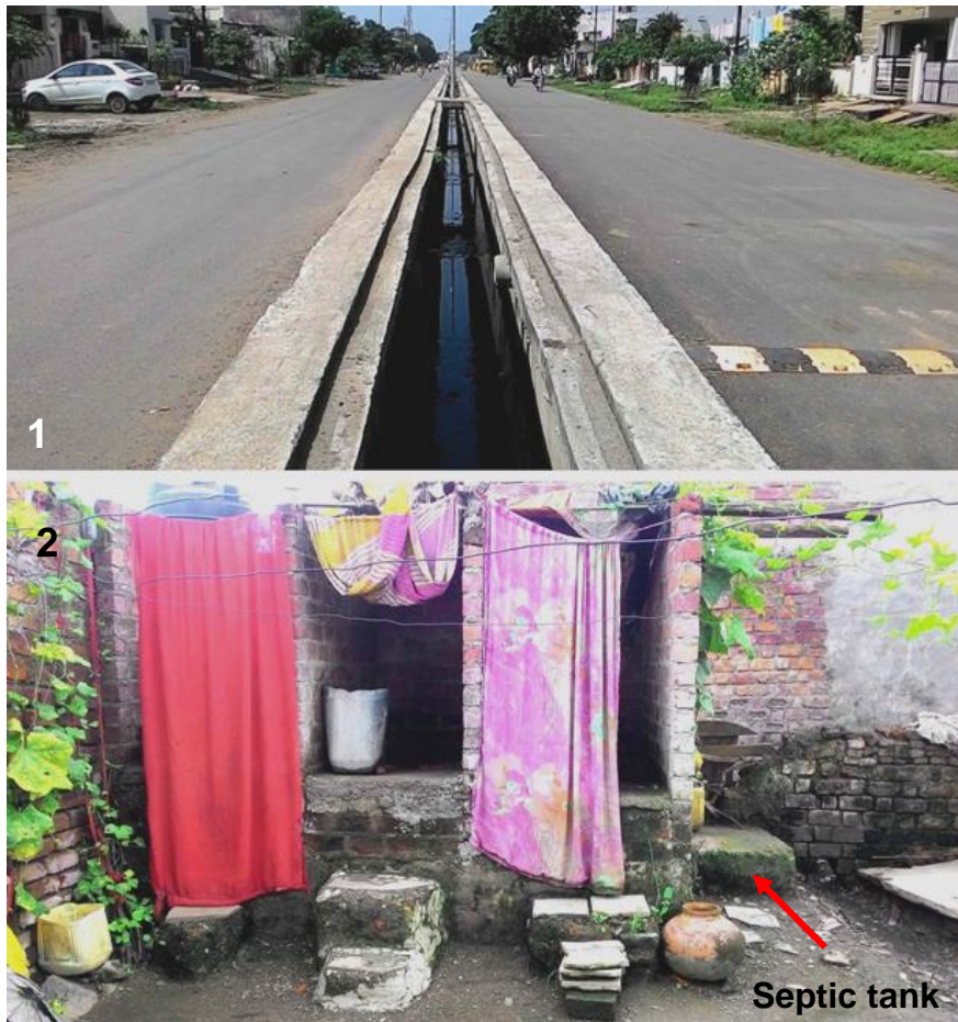
Figure 5: Trunk sewer and containment system (Source: Shantanu/CSE, 2015)
