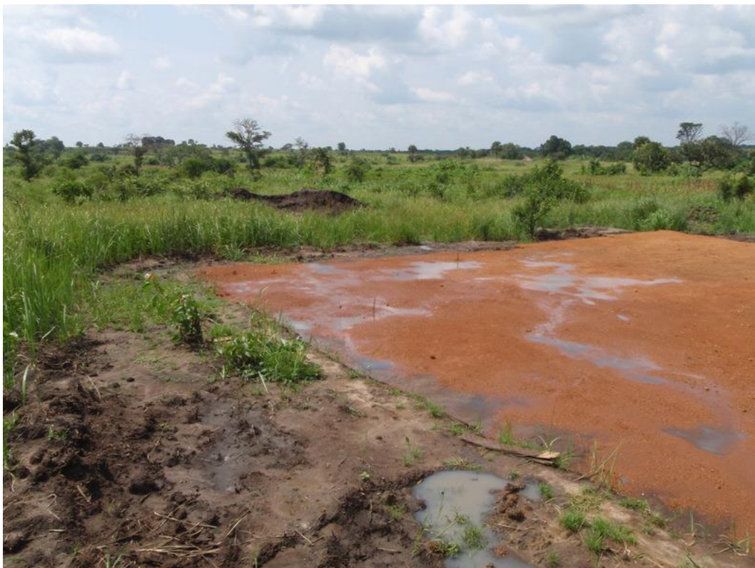
Figure 2: The future sludge drying beds (source: GIZ)
