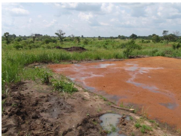
Figure 2: Construction site of future sludge drying beds (Source: GIZ 2015)
