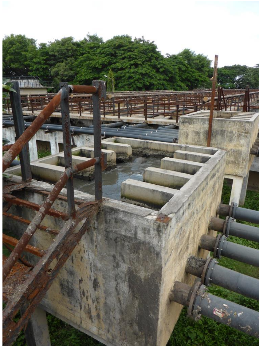
Fig. 2: Upflow Anaerobic Sludge Blanket (UASB) facility at Tapovan WWTP (August 2015, L.Roeder)
