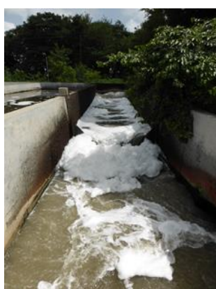
Figure 1: Foam formation in treated effluent of Tapovan wastewater treatment plant (Roeder 2015)
