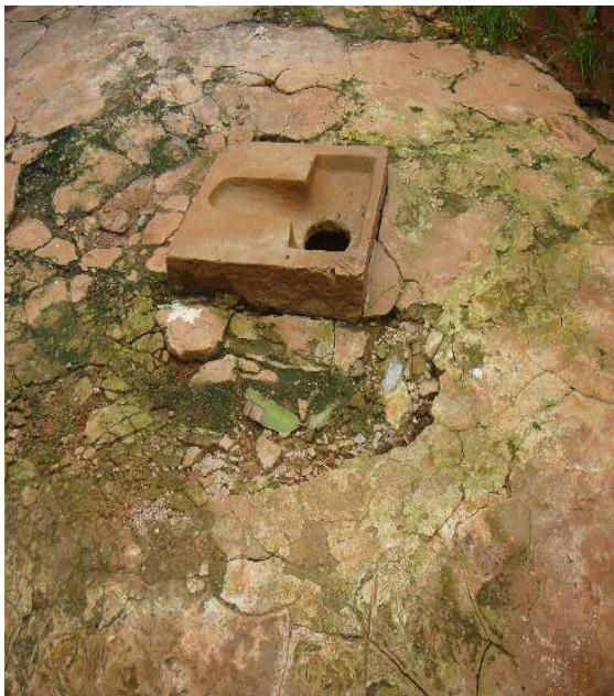
Figure 6: User interface (left) and wall of unlined pit in Bignona, Senegal (H2O and I&D, 2014)
