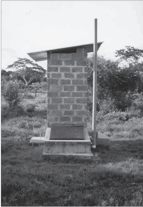
Photograph 5.1. Solar urine-diverting latrine in El Salvador
