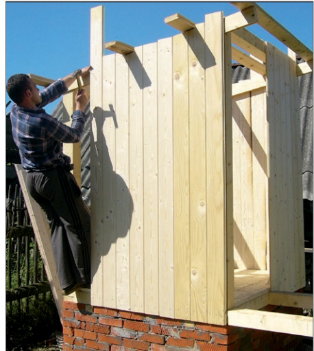
Framing the toilet room with 2 cm thick wooden slats
