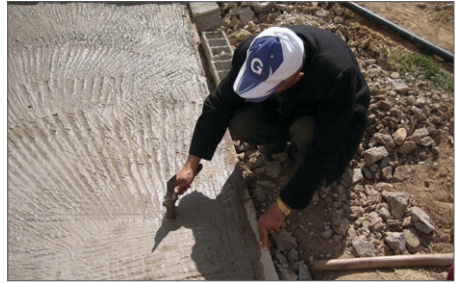
Laying floor slab with high quality concrete
