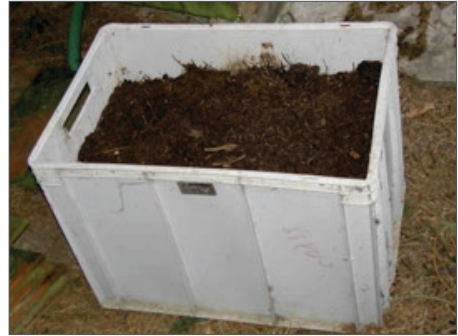
Filled box of a single vault urine diverting dry toilet
