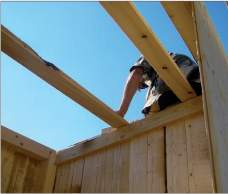
Constructing roof with wooden slats
