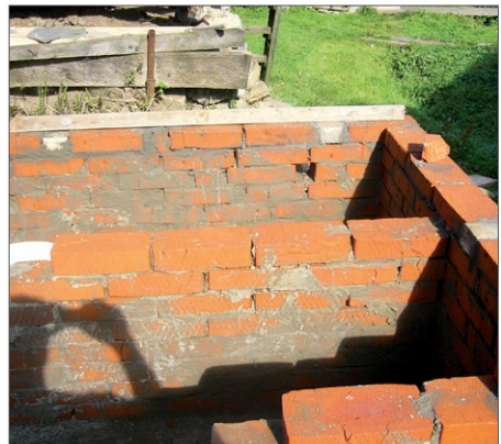
Faeces vaults built on top of floor slab
