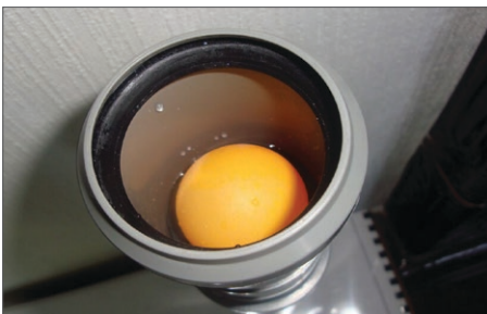
Solution 2: table tennis ball installed below the urinal. Photo from Dima Mamaliga, Apasan, Moldova
