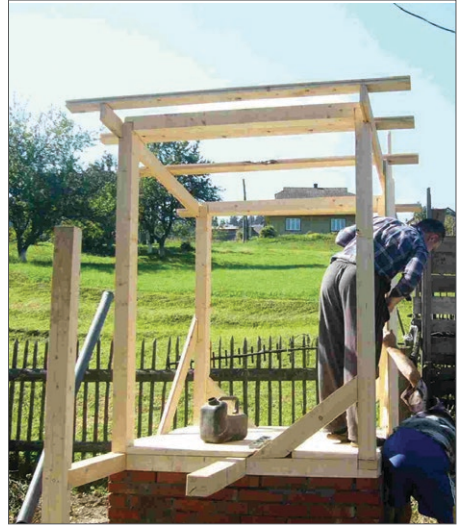
Constructing a frame
