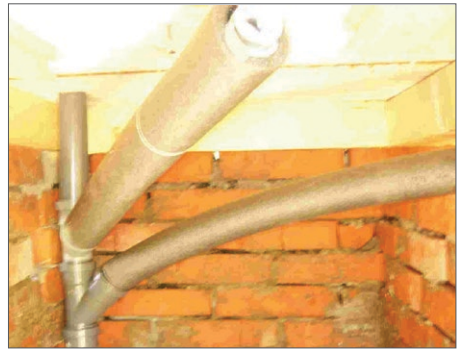
Good example of pipe installation with insulation for colder climates
