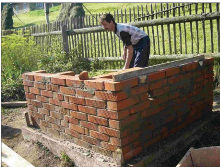
Building dividing wall with bricks
