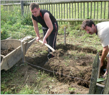
Excavation for the foundation
