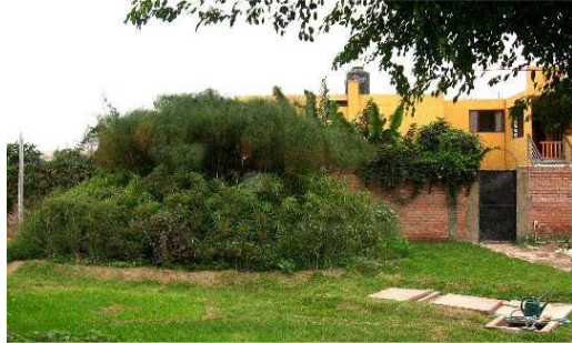
Fig. 19: Constructed wetland (reed bed) for greywater treatment planted with two species of Papyrus, after 1 year of operation.
