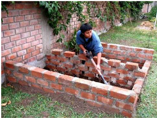
Fig. 7: Spreading of the retained solids from the filter bag, after 6 months (see Fig. 6) on the vermicomposting bed on a concrete slab
