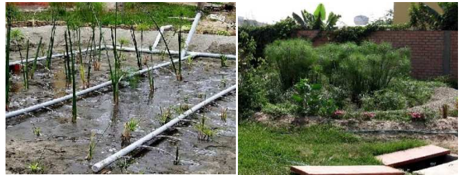
Fig. 5: Vertical flow constructed wetland for greywater treatment during pumping (a day after planting and before the protection of the distribution pipes with a 10 cm gravel layer) (left) and after two months, with storage tank for irrigation of treated greywater (right).
