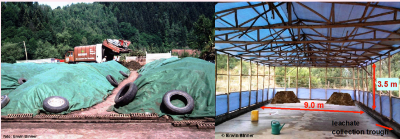
Figure 6. a) Windrows covered by geo textile b) example for a rotting platform roofed by shed.
