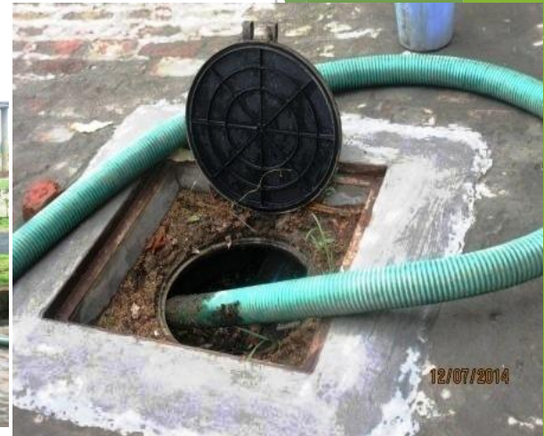
Desludging of system
