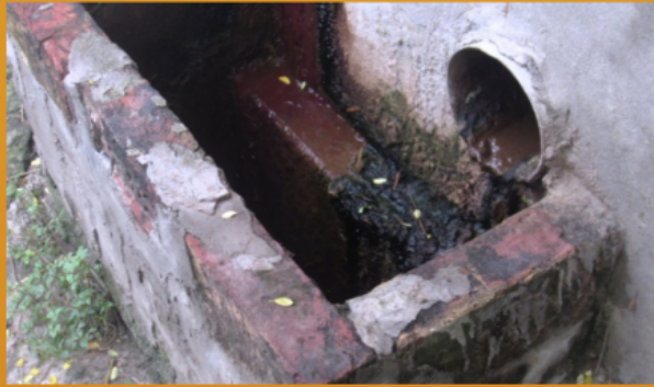
Connection to open drain
