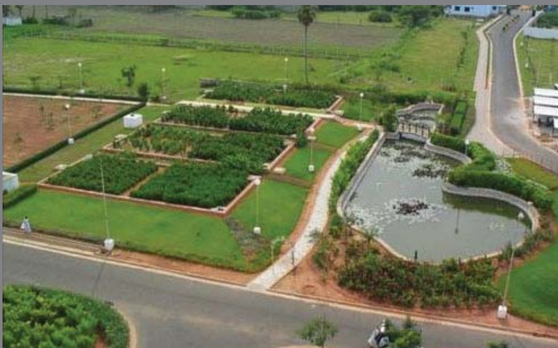
DEWATS system maintains aesthetics of the campus
