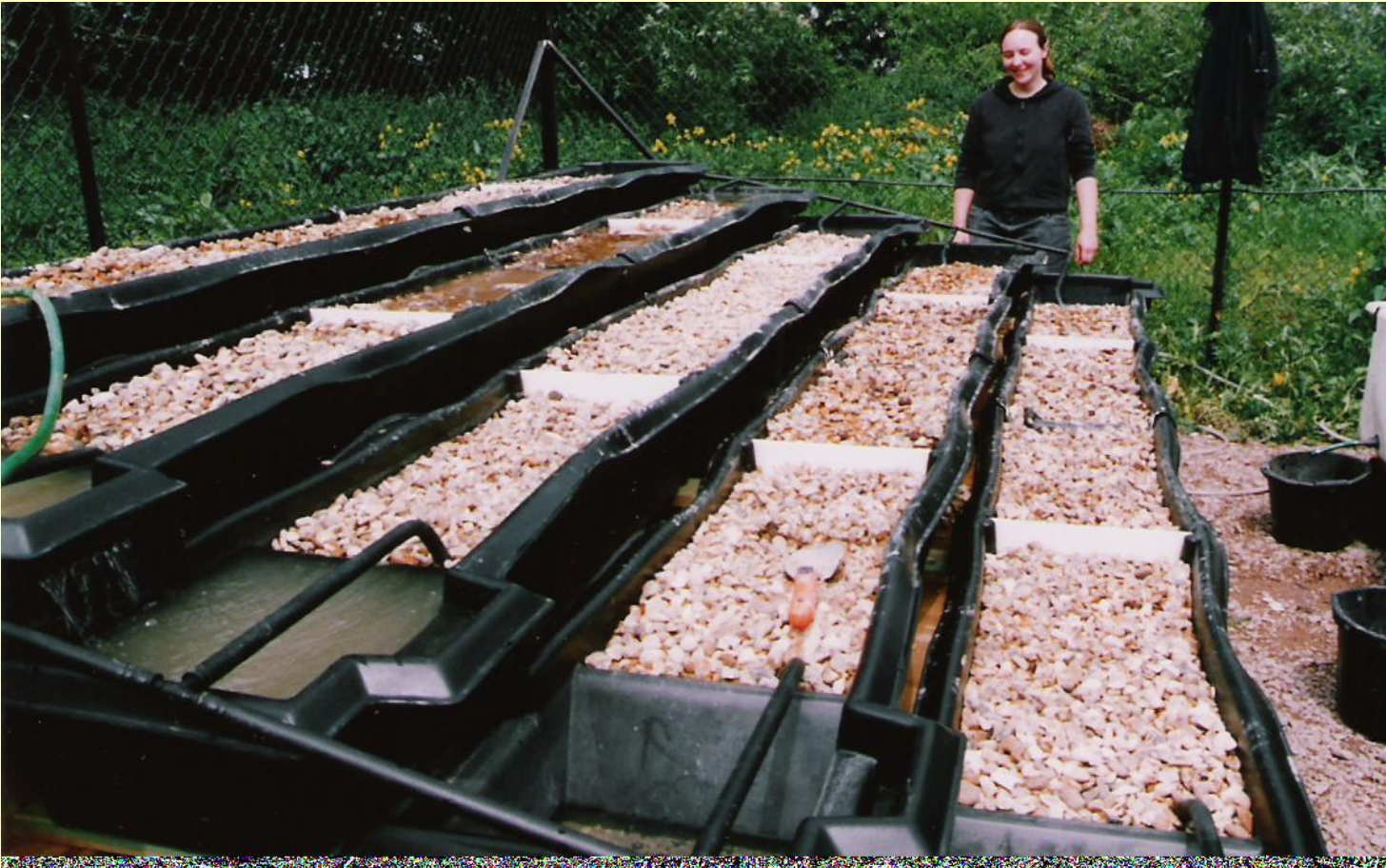
Construction of GROW rig at Cranfield University May 2004 – showing troughs filled with gravel
