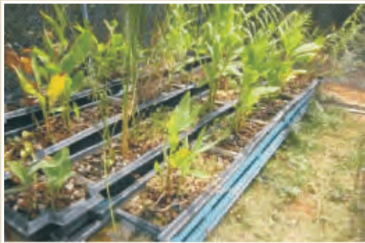
Grey water Recycling system at IIT, Madras SARASWATI Project
