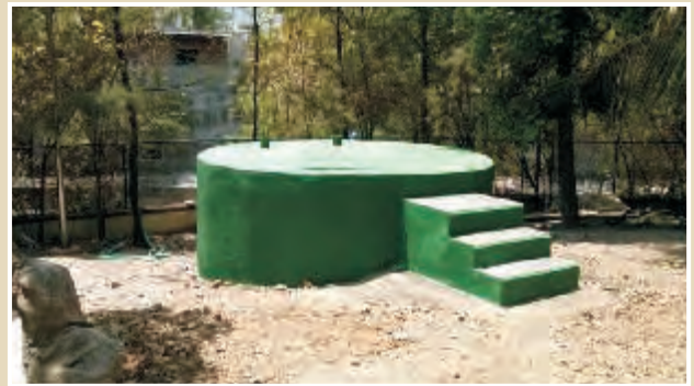
Intake Well NaWaTech Project
