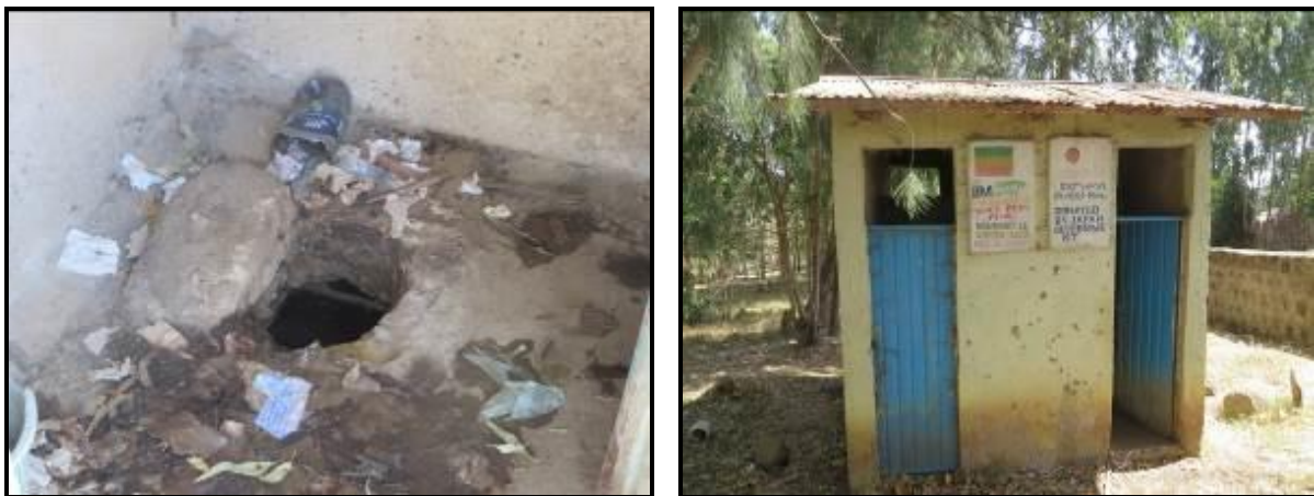
Figure 3: Inside and outside of a public latrine (photo credit: Oscar Veses)
