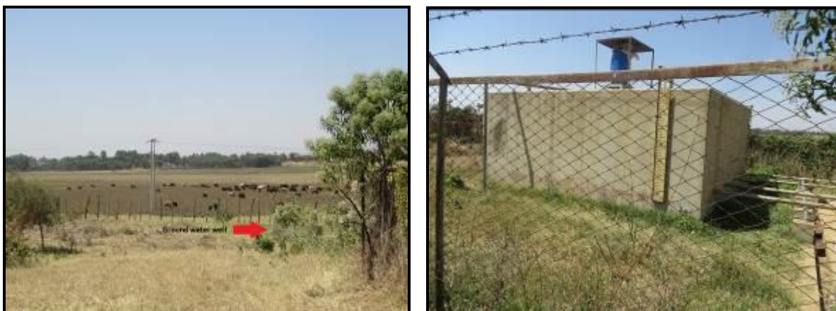
Figure 12: a) Well for water supply surrounded by cattle rising. b) Reservoir with chlorine dispenser (photo credit: Oscar Veses).
