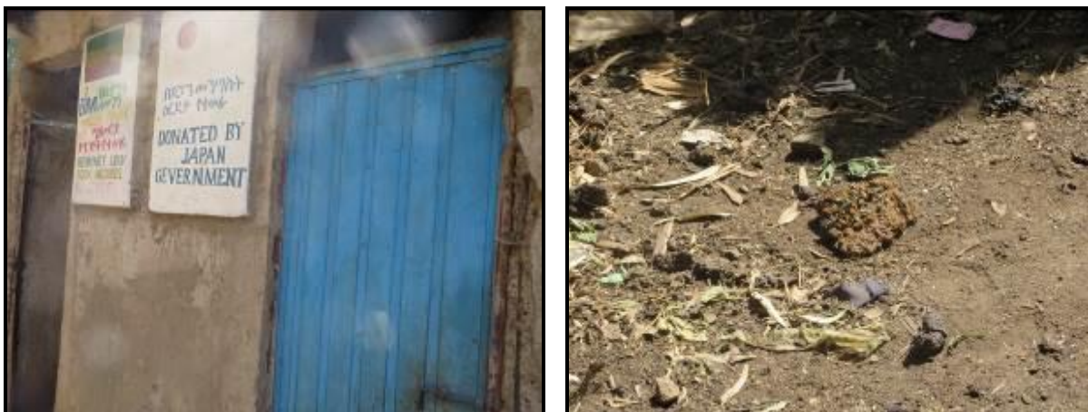
Figure 4: a) Front of a public latrine which is not emptied when full. b) Outside of the latrine with some faecal matter in the ground (photo credit: Oscar Veses).
