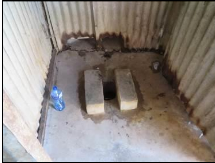
Figure 5: Inside of a latrine (photo credit: Oscar Veses).
