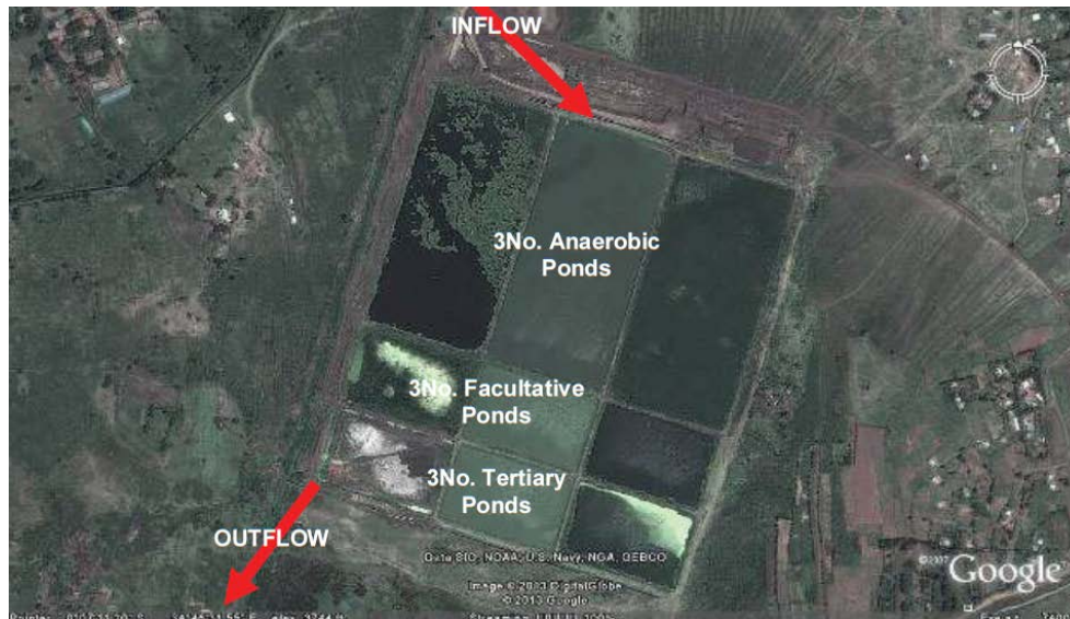
Figure 4: Nyalenda STP pre- rehabilitation (World Bank, 2013)
