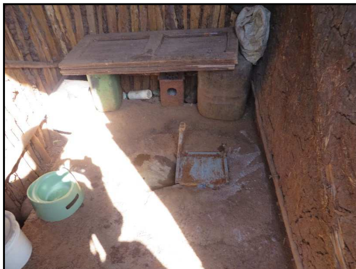
Figure 5: Inside of an improved latrine in Holleta (photo credit: Oscar Veses).
