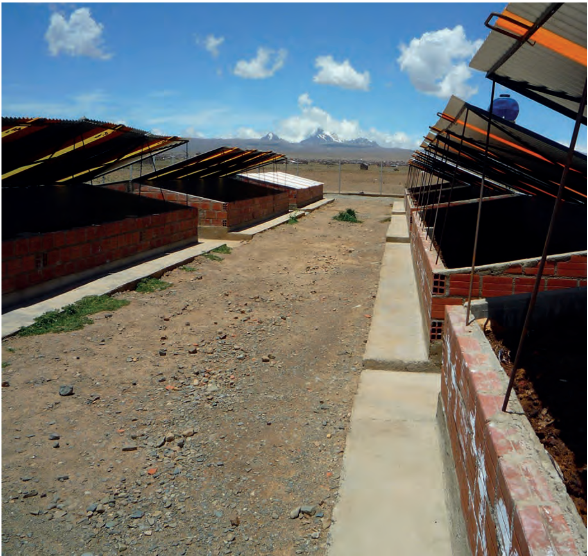
Faeces composting for agricultural reuse in a project in El Alto, Bolivia. Urine and faeces are collected separately using urine-diverting dry toilets. Greywater is applied to household constructed wetlands. Photo: Kim Andersson
