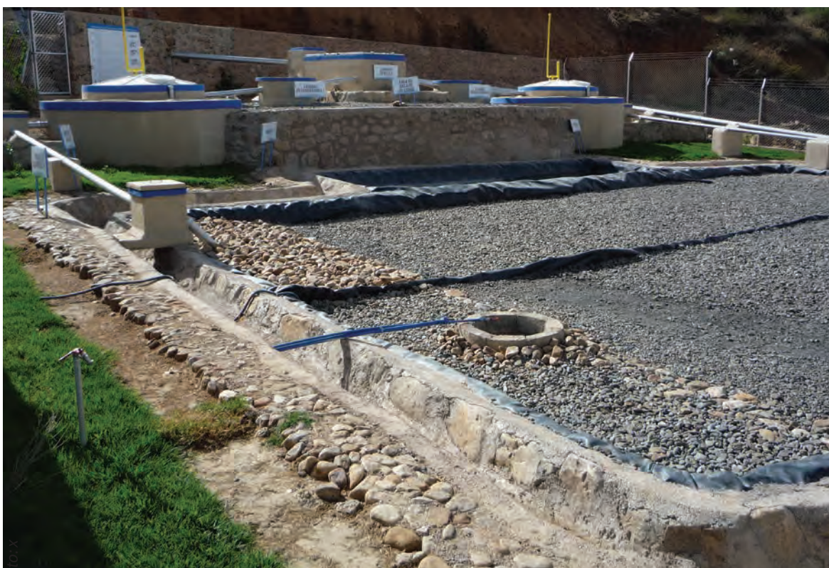
Decentralized wastewater treatment plant with constructed wetland, Cochabamba, Bolivia. Photo: Kim Andersson
