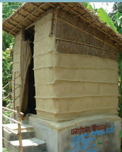
This project in Bihar, India, tackled the financing issue by providing the concrete substructure for flood-resistant toilets, while households were responsible for building the superstructure. Photo: Kim Andersson
