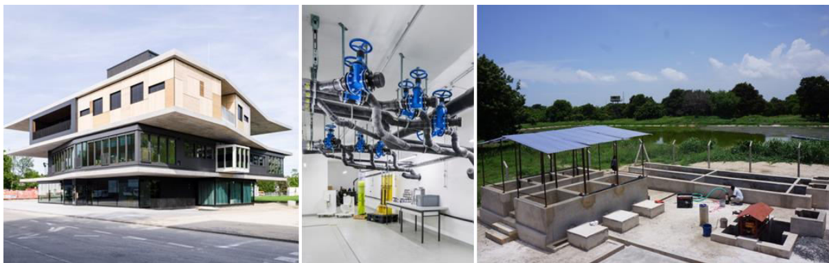
Figure 1. Left image: The NEST building with a residential research module installed on the second floor; Centre image: Pipes leading into the WaterHub laboratory, separately transporting FS, urine, and greywater to research stations; Right image: The FS dewatering facility in Dar es Salaam.
