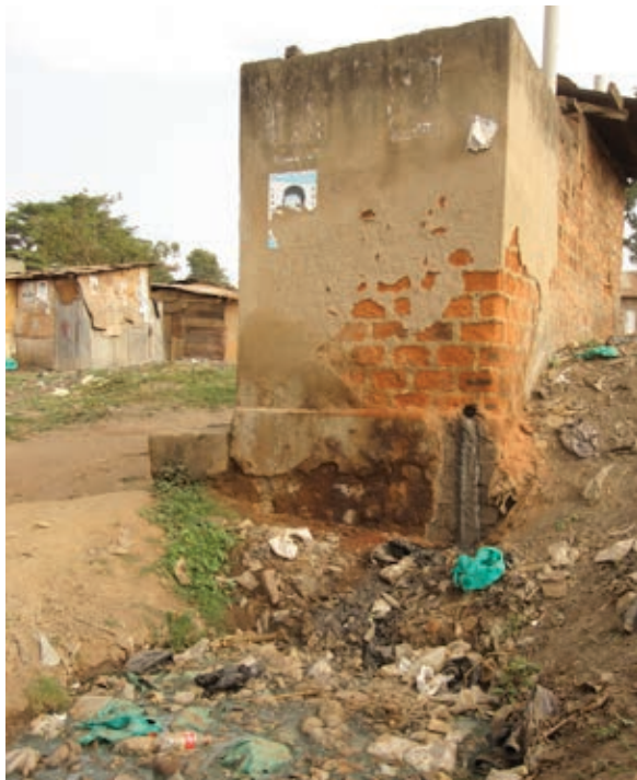
Figure 2: Typical pit latrine
