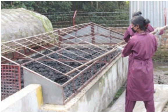
Picture 2: Dry sludge being removed from the drying bed by operators
