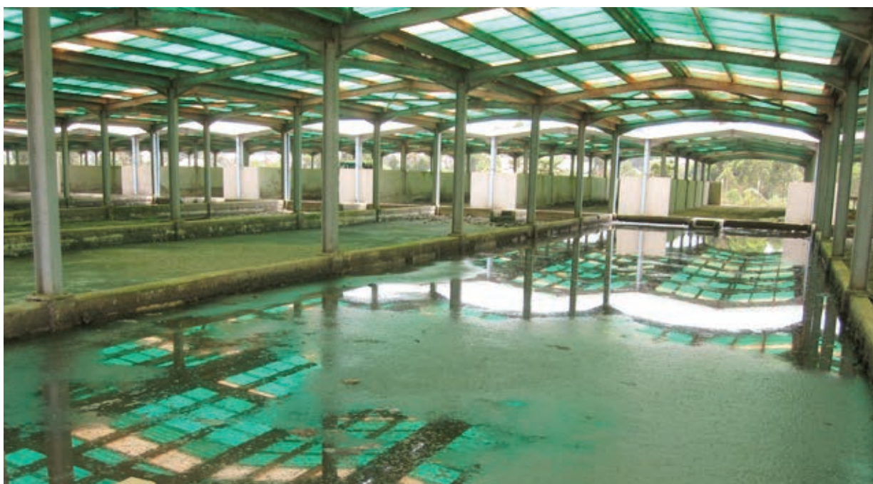
Figure 3: Sludge Drying at Lubigi Treatment Plant
