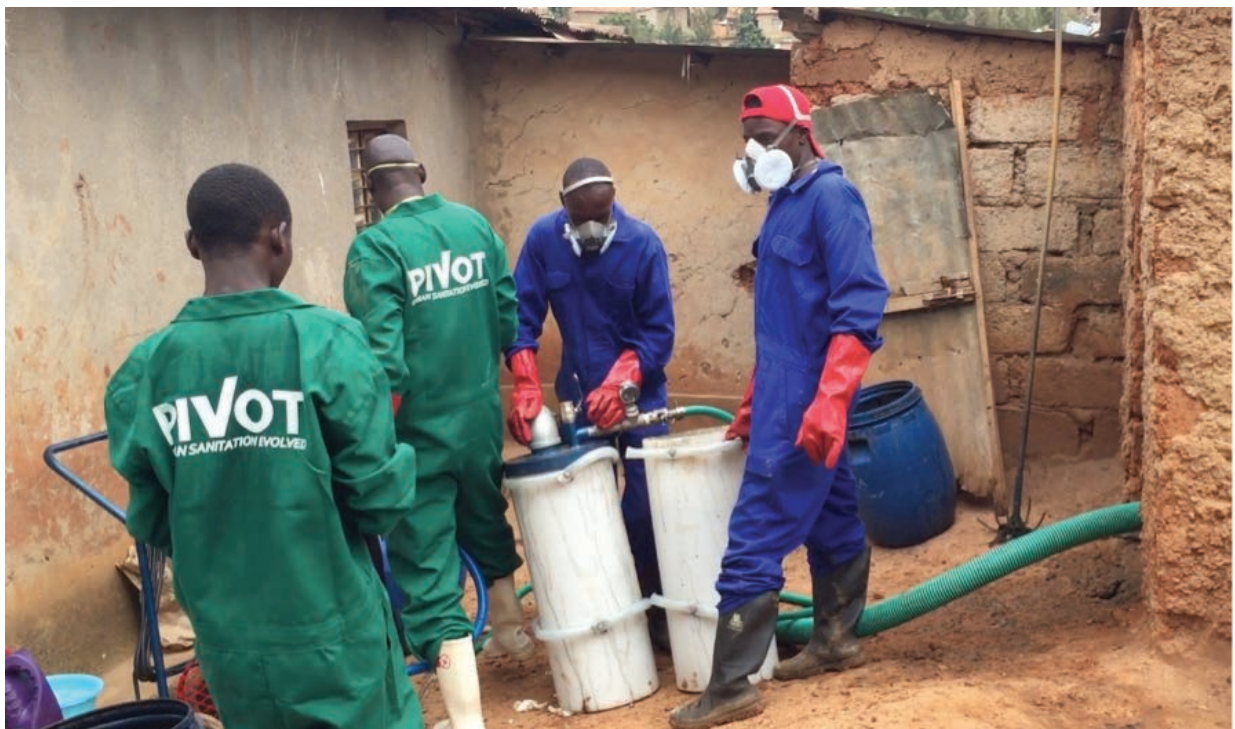
Figure 2. Pit Vidura team emptying a pit in the Gitega sector of Kigali.
