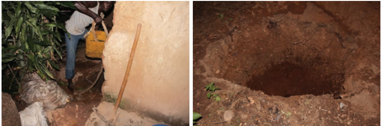
Figure 1: Emptying observation. a. Pit excavation of 10-meter burrow hole using one jerry can; b. Dumpsite located ~30 meters from the pit.
