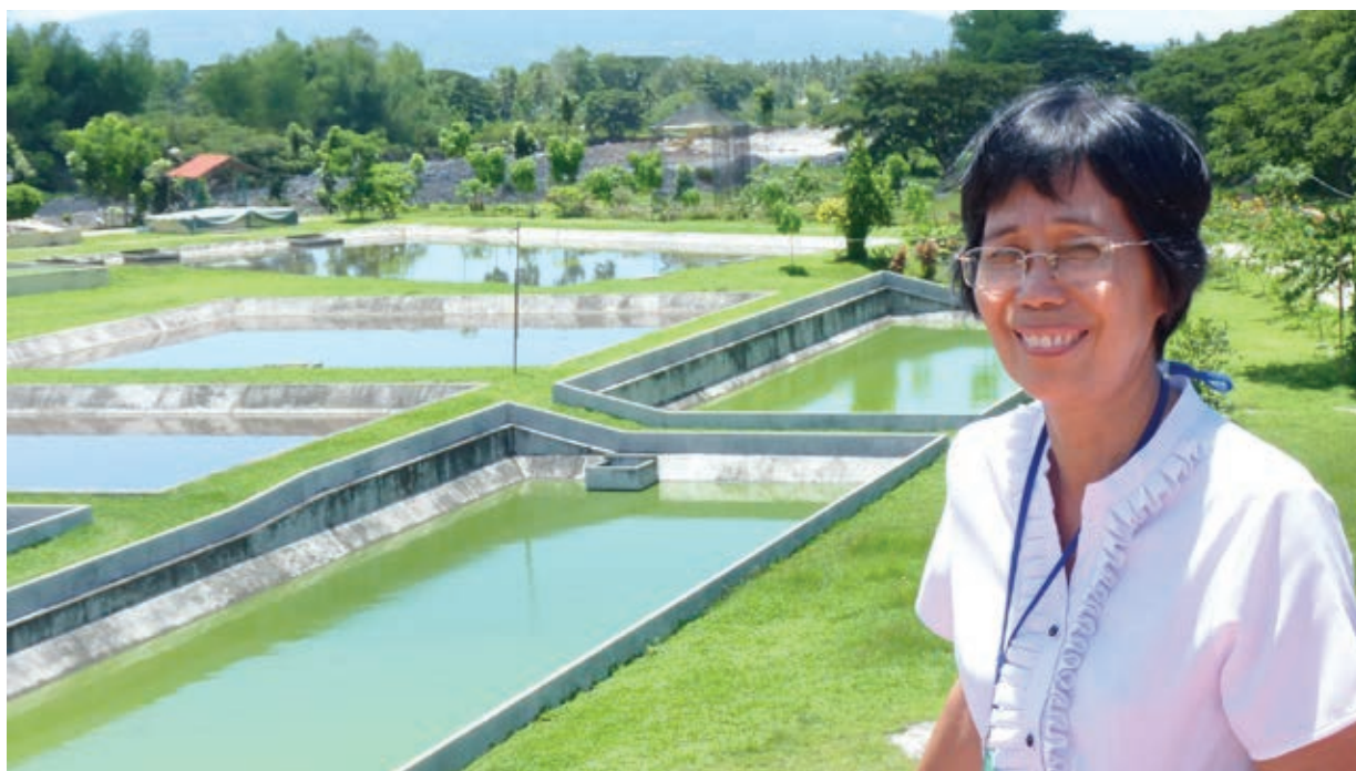
Figure 1: Dumaguete Septage Treatment facility uses waste stabilization ponds, constructed wetlands and sand drying beds. Josie Antonio, Chief Planning Officer 2003–2011 in foreground.
