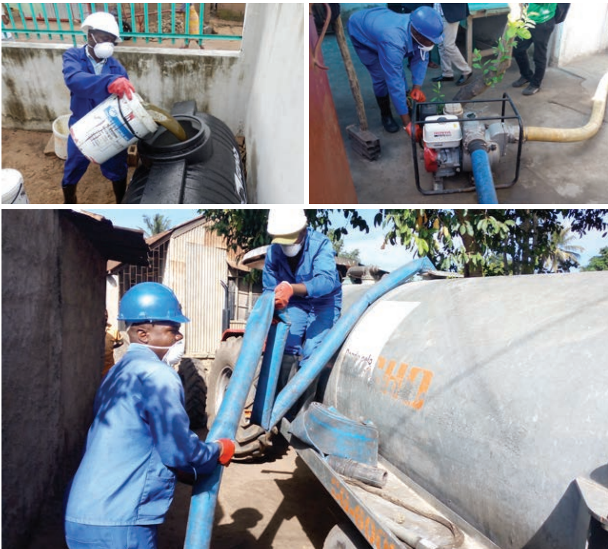
Figure 3: Small business desludging operations with a trash pump and small tankers
