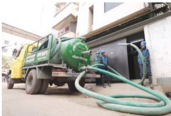
Figure 5: SWEEP team prepare to empty a customer's tank
