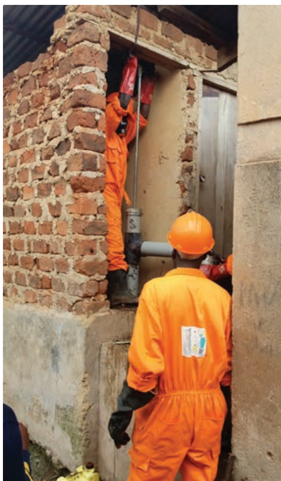
Figure 6: Using a Gulper to empty a pit latrine
