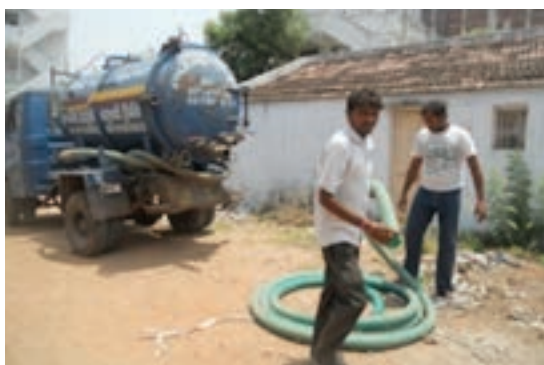
Desludging operators have no safety equipment for desludging septic tanks
