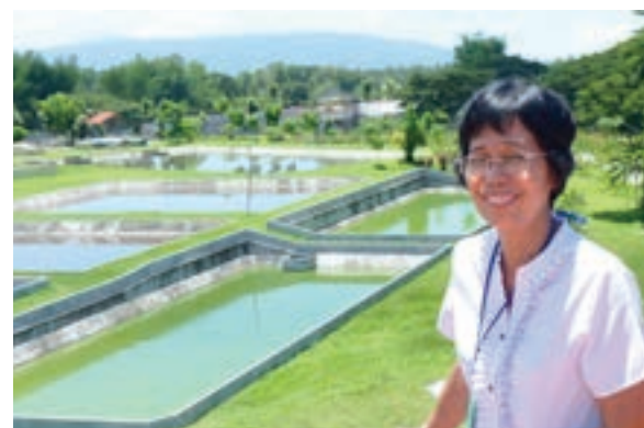
Figure 3: Waste Stabilization Ponds at the Dumaguete City Septage Treatment plant. Josephine Antonio, Chief Urban Planner at the time of construction.
