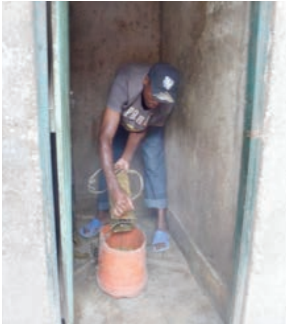
Figure 1: Manual emptier emptying a pit latrine with a bucket ©GIZ/Doreen Mbalo
