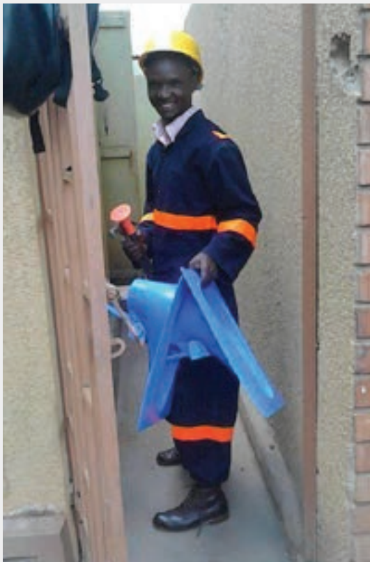
Figure 8: Forever Sanitation proprietor John Busingye with Sato pans for installation
