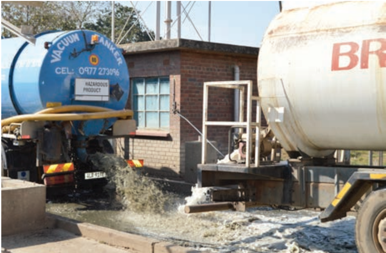
Figure 2: Tankers discharging faecal sludge
