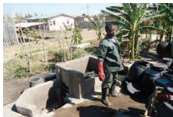
Figure 3: Kanyama faecal sludge treatment plant
