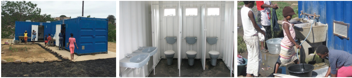
Figure 8: Photographs showing components of a community ablution block in an informal settlement
