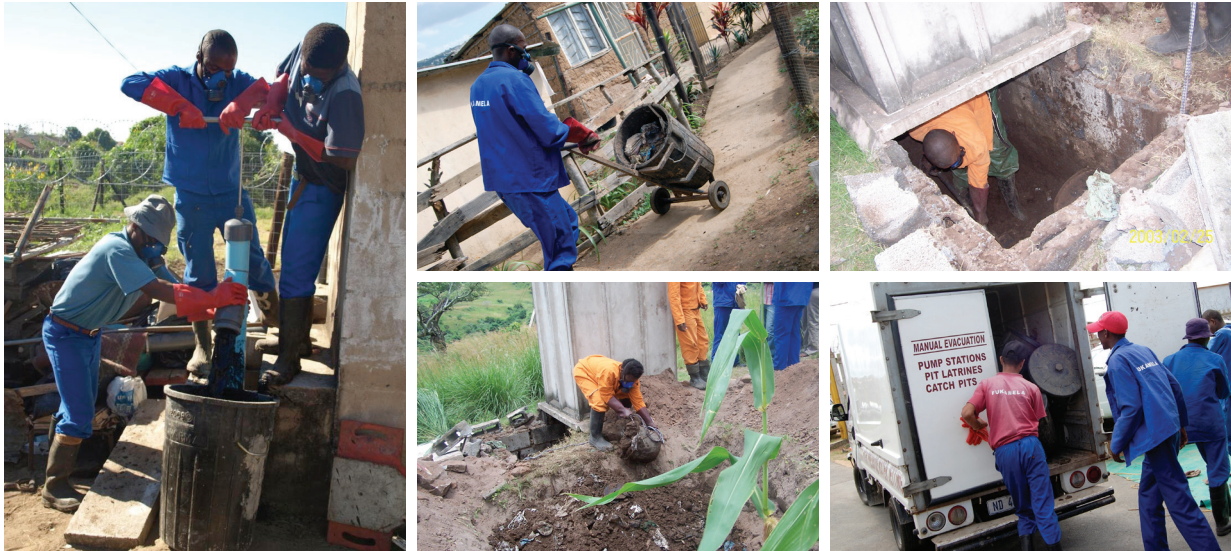
Figure 2: Photographs showing emptying and transport of waste from VIP toilets
