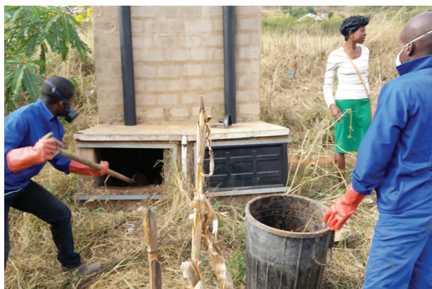
Figure 6: Photographs showing the components of a urine diversion toilet and emptying activities
