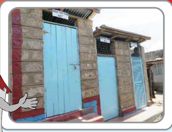
TOILET "A" AFTER REHABILITATION
