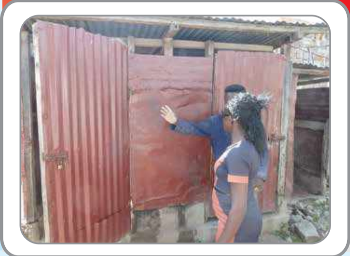
TOILET "A" BEFORE REHABILITATION
