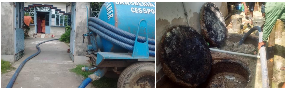
Figure 4: BM vacuum tanker used for emptying septic tank/twin pit system (Source: Anil/CSE, 2016)
