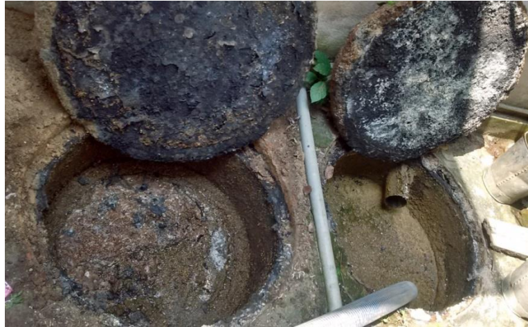
Figure 3: Twin pit latrine (Source: Anil/CSE, 2016)
