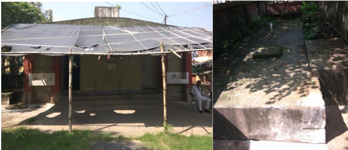
Figure 27: Public toilet connected to ST near Haneswari Temple (Source: Aishwarya /CSE, 2016)
