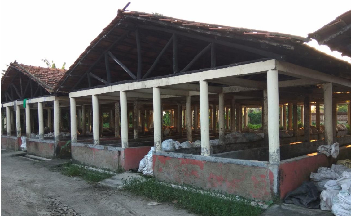
Figure 145: Sludge drying facility at FSTP (Source: Anil/CSE, 2016)
