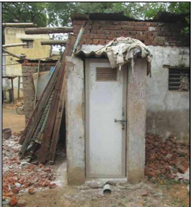
Figure 7.6: An unused household latrine used as a store (left) and an inappropriate outlet for sewage from a household latrine (right)
