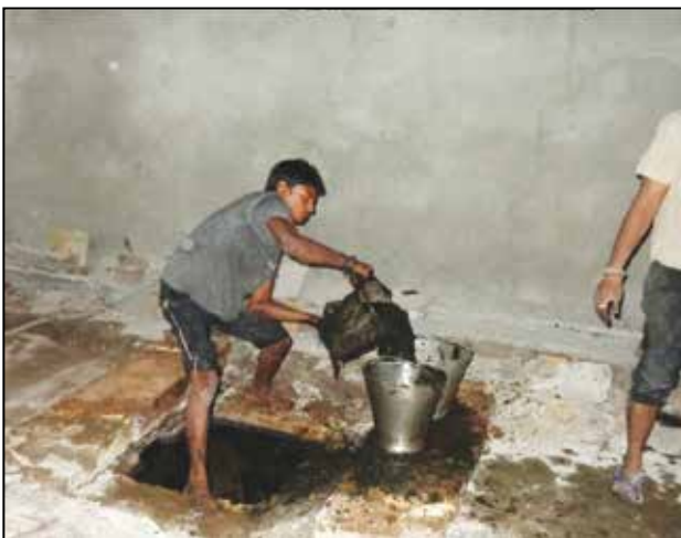
Figure 7.5: Manual emptying of a soak-pit (left) and disposal of sewage into an open drain adjacent to water facilities
