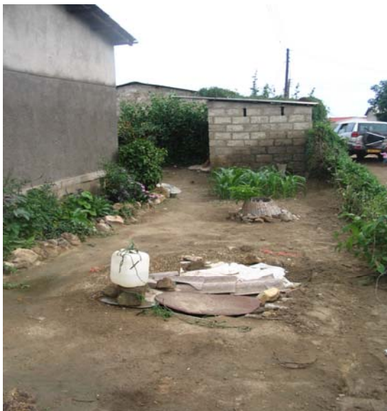
Figure 4-13 Pit toilet in the background and shallow well in the foreground (distance apart is approx. 15 m) on plot in John Laing.
