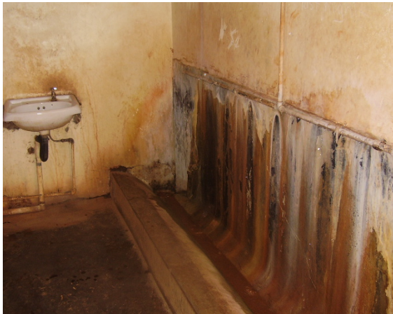
Figure 4-3 Urinal in the boys' toilet at the old govt. school.
