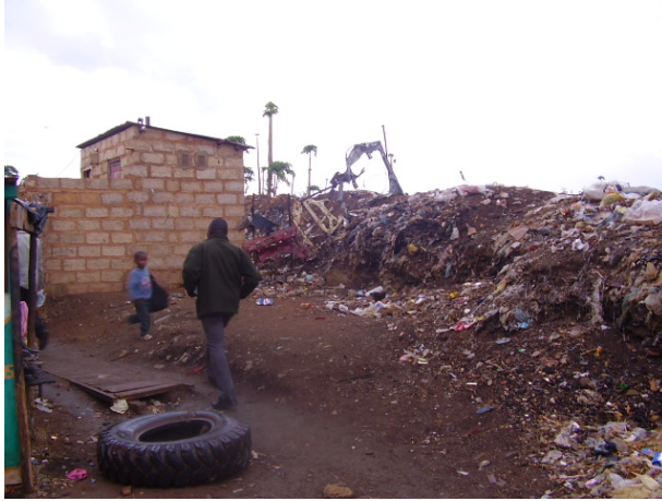
Figure 4-5 Public pit toilet at the Bauleni market place (notice the uncollected solid waste pile !!)
