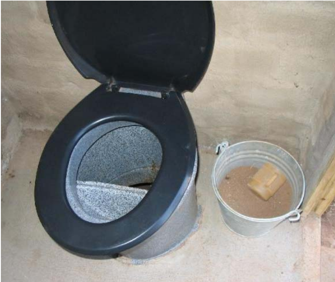
Figure 2-8 Dry Urine diversion toilet pedestal with bucket of sand or ash (Münch, 2005)
