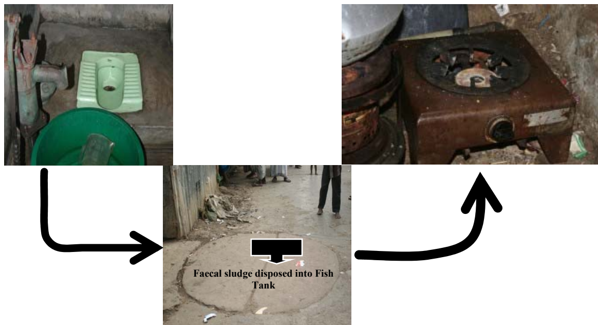
Figure 2-12 Photo schematic of sanitation layout at household level in Baunia Bandh baste, in Dhaka, Bangladesh. Source: (Islam, 2006)
