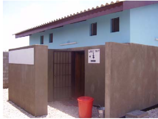
Figure 4-10 A donor financed public fee paying toilet and shower near a market place in Chawama. This system is waterborne with septic tanks and soak-away.
