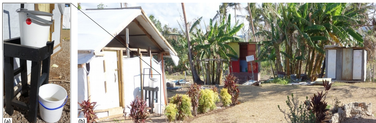
Figure 38: A hand washing facility (a) is placed in front of each of the three temporary classrooms (b, left) which were put up after the main schoolhouse was damaged during TC Pam. Further the Composting Toilet in red (b, middle) and two of the four Pour-Flush Toilets (b, right) are depicted.
