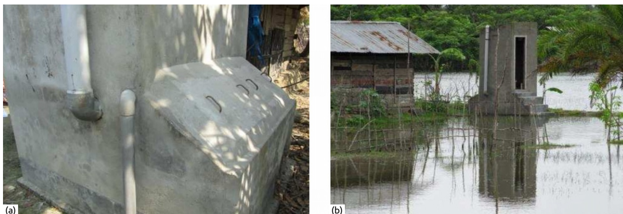
Figure 24: This UDDTs have been successfully implemented in Bangladesh for flood heights up to 0.9 m. Vault doors out of concrete are used due to better corrosive resistance (a). The toilets proved to be working during cyclone Aila in May 2009 (b) (Delepiere, 2011. p. 4, 6).
