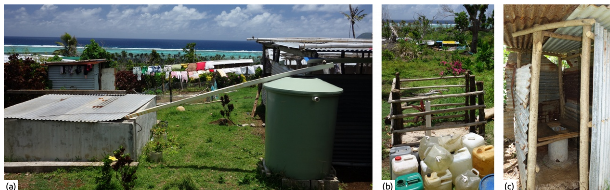
Figure 47: The view from Makatea including a Dry Toilet behind the concrete storage tank on the left, and another tank out of fiber-glass on the right hand side is shown in (a). One of the four lockable taps with multiple jerry cans used to obtain drinking water is depicted in (b), and (c) shows a Dry Toilet from the village.
