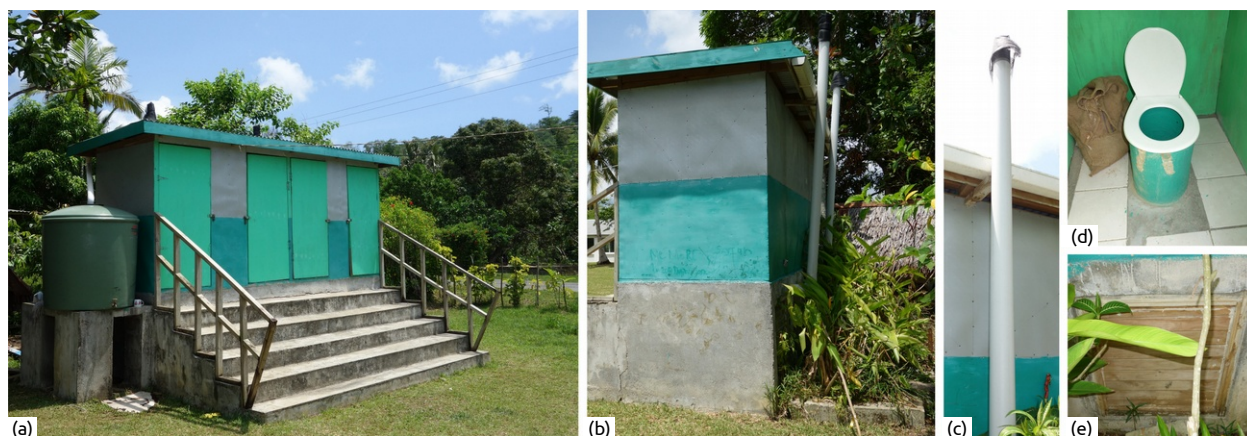
Figure 43: Composting Toilet at a church in Solway with separated toilets for men and women, and a tank for rainwater storage (a). A planted infiltration bed was implemented in the back (b). One vent pipe aerated both vaults. It protruded about 50cm above the roof. A fly screen was fitted at the end, but a rain cover was missing (c). The toilet cubicles were clean and partly tiled, bulking material was available (d). All four vault doors were in good order (e).
