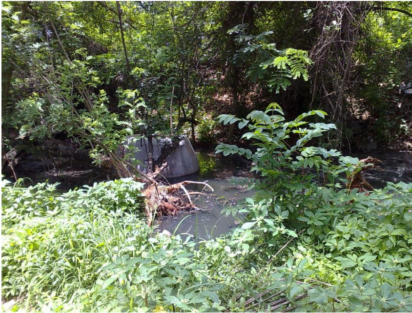
Sewage water flowing out from Manhole in Mysore University area
