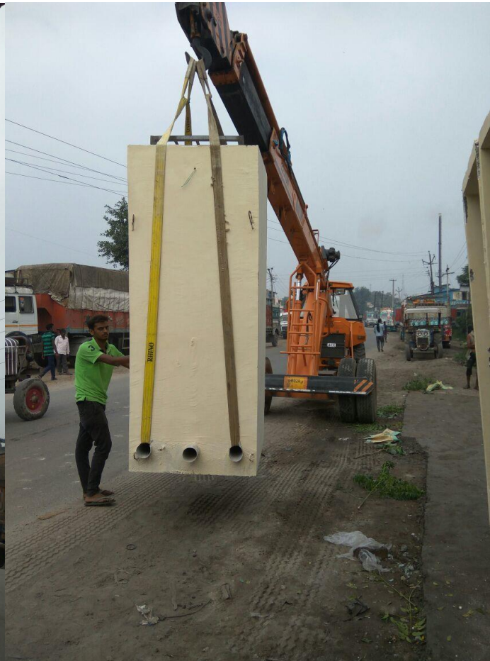
2. Lifted using crane and placed onsite
