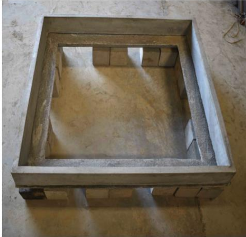
1. Lay the foundation on an even surface
