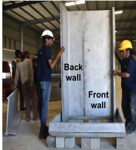
2. Place 1 front and 1 back wall on ring
