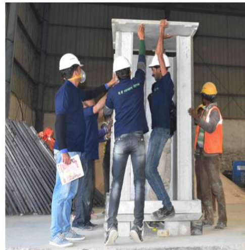
5. Place the roof and close the locks
