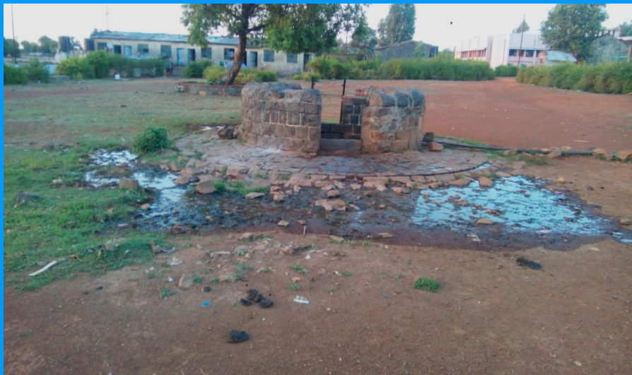
Water logging with no proper drainage
