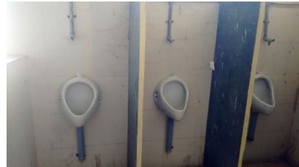
Boys Urinal Repaired: Bhamragad PO
