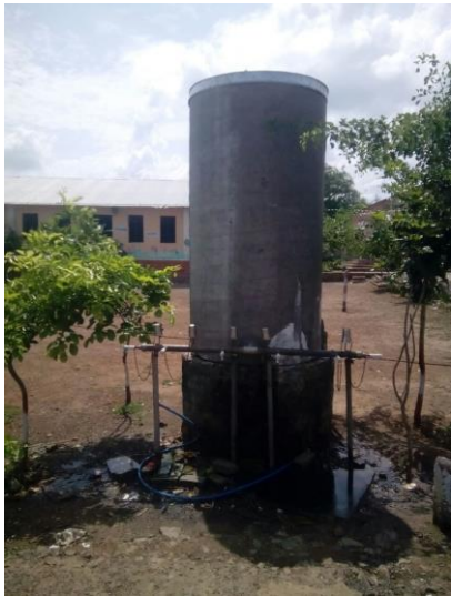
Water tank with taps :AKOLA PO
