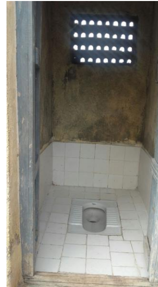
Girls Toilet Repaired with new toilet seats and flooring: Solapur PO
