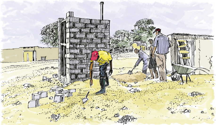
Figure 6. A VIP latrine under construction
