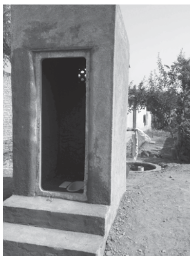
Figure 1 Newly constructed Tiger Toilet, showing the tank and collection pipe in the background
