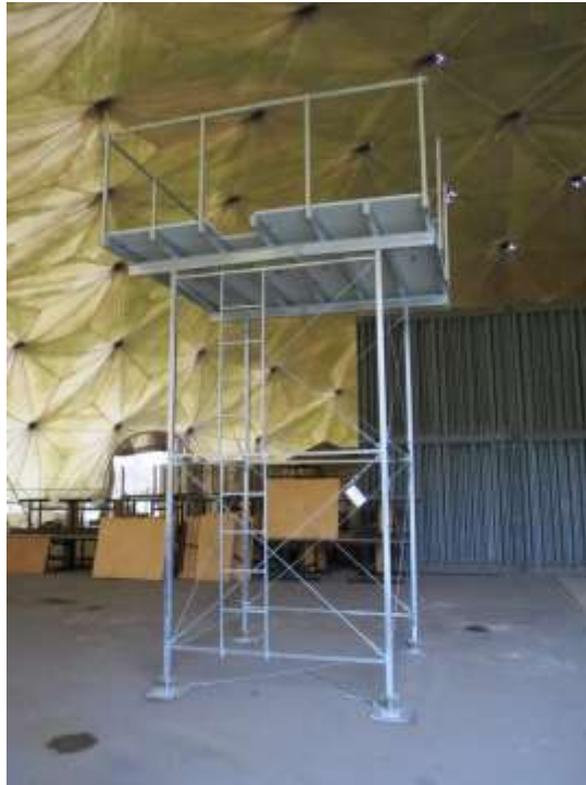
Figure 70: Picture of the assembled prototype of the water tower.
