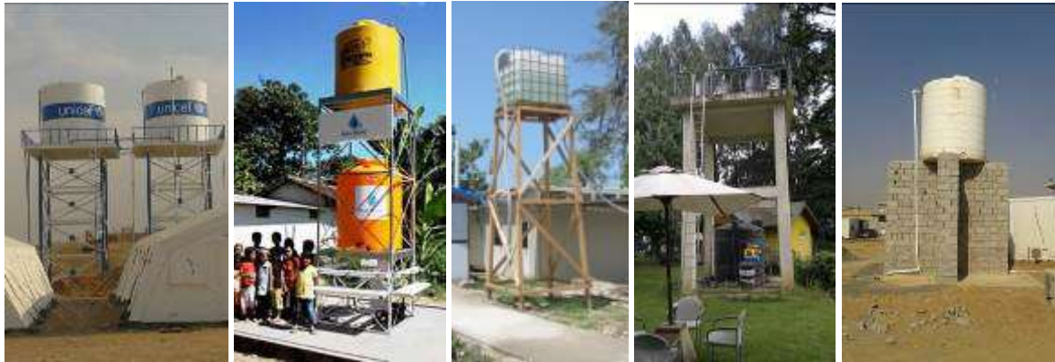
Figure 47: Examples of material use in water tower structures (from left to right: steel, aluminum, wood, concrete, brickwork).
