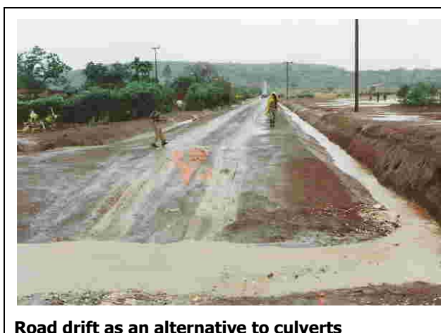
Road drift as an alternative to culverts
