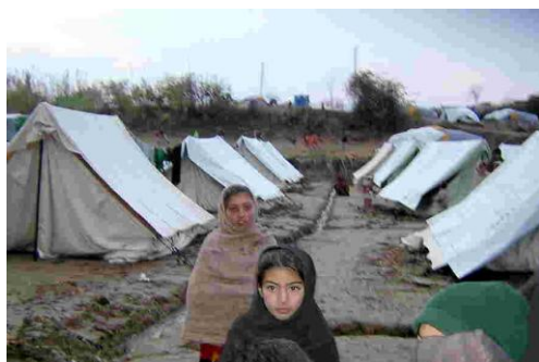
Simple earth drains being constructed to reduce the muddy conditions around the tents in Jabba tented village, IDP camp in Pakistan
